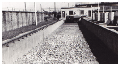
Test section of flexible pavements in Tišnov
