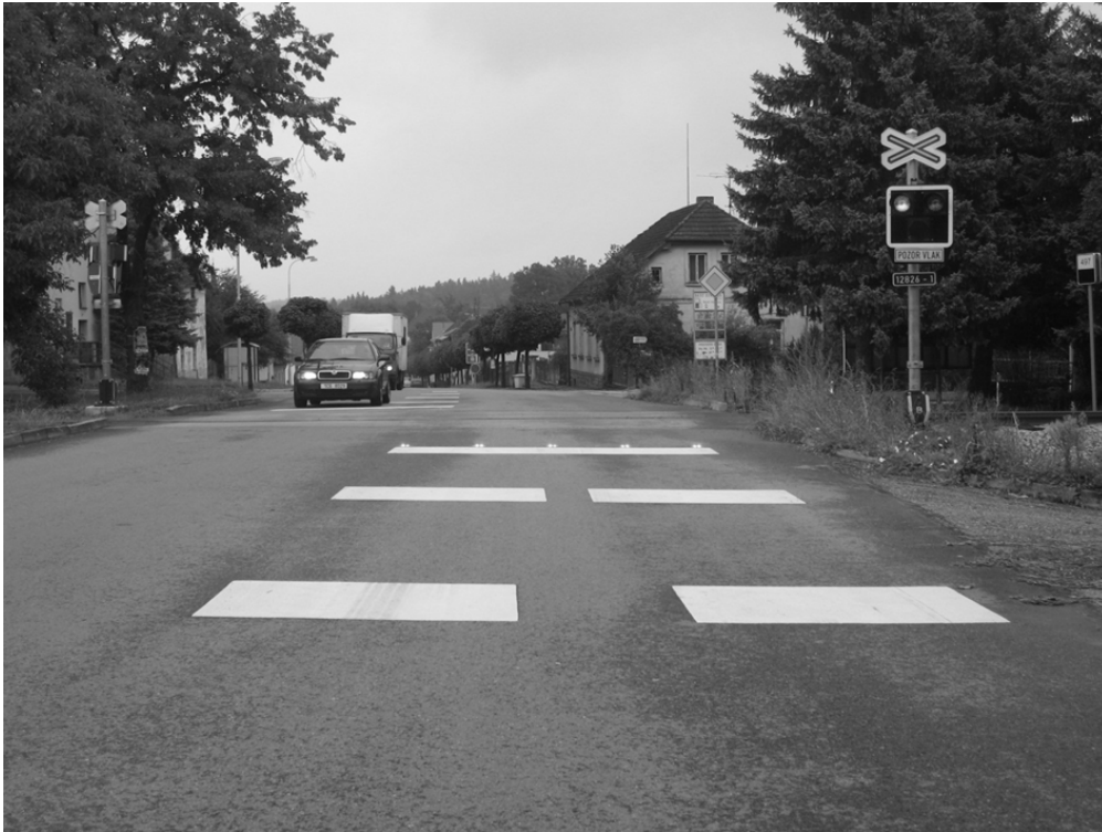
Figure 1: Light barrier in Nová Včelnice.
